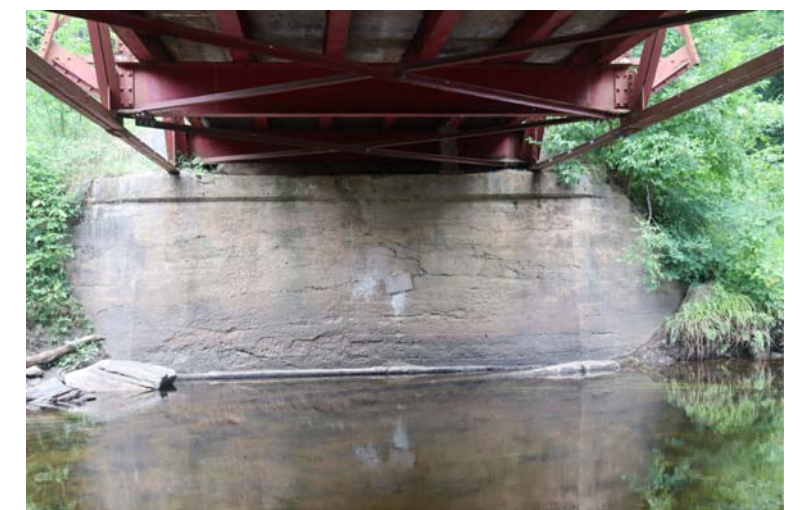
TYPICAL ABUTMENT & WING WALLS
