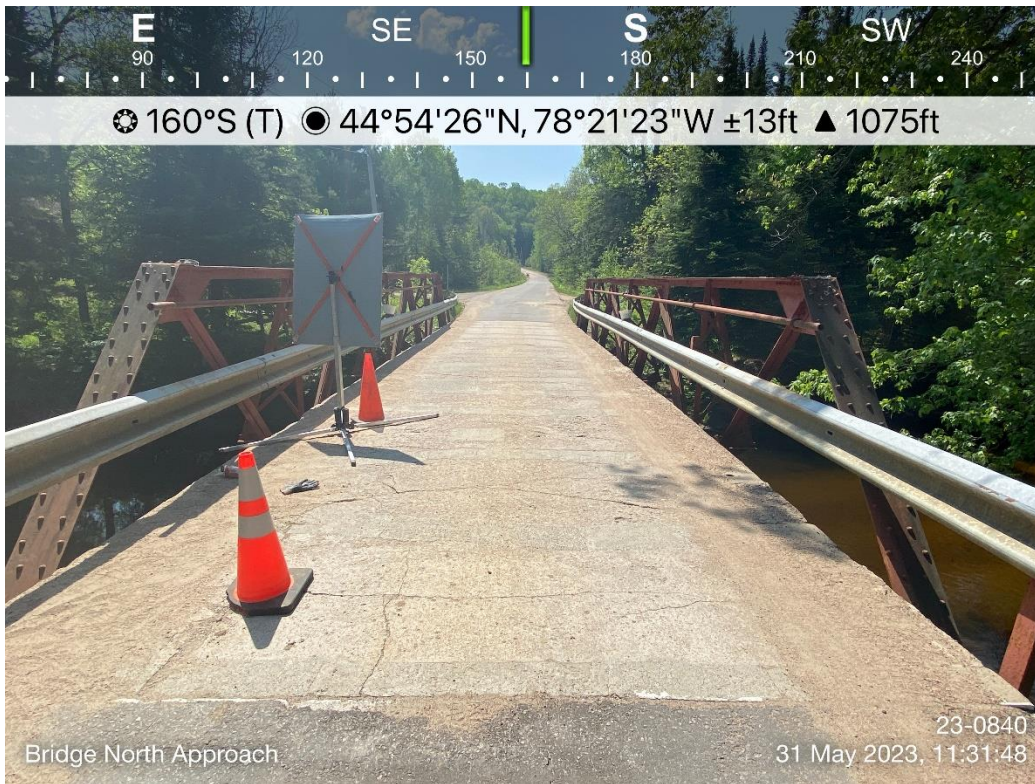
Photo 10: Bridge north approach. Photo taken face south.
