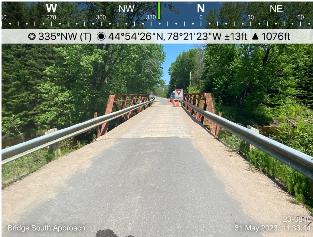
Photo 9: Bridge south approach. Photo taken facing northwest.
