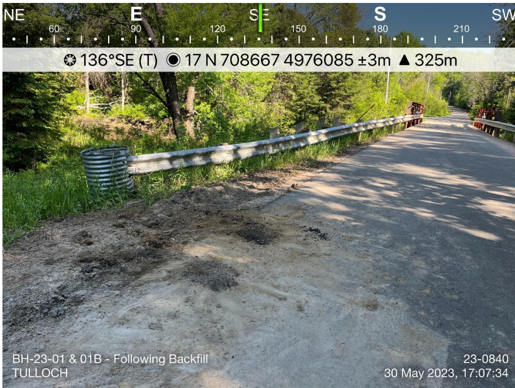
Photo 2: BH-23-01 following completion of backfill. Photo taken facing southeast.
