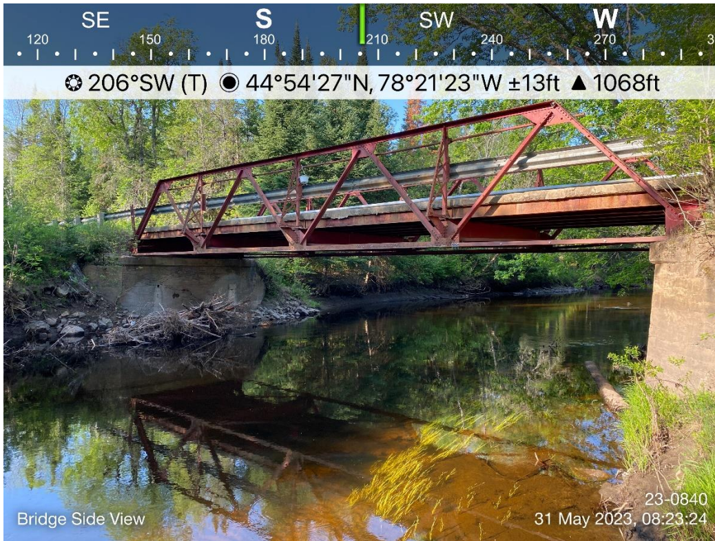
Photo 7: View of bridge and river banks facing southwest
