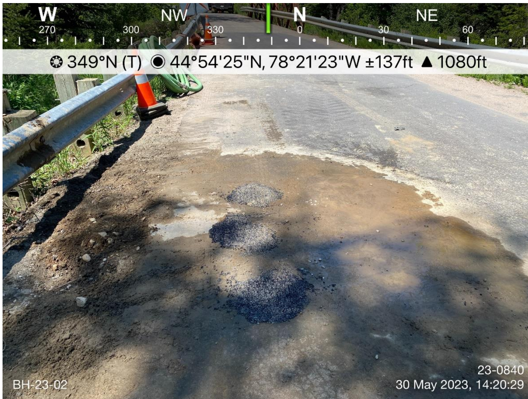
Photo 4: BH-23-02 following completion of backfill. Photo taken face north.
